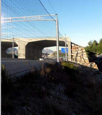
Photo 1 - Detail of the net that covers the A7 in the vicinity of the bat shelter (© Miguel Angel Monsalve)
