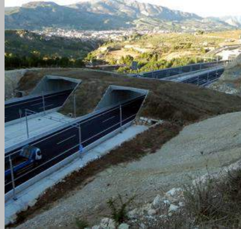
Photo 2 - Overpass details (© J. Juste)
